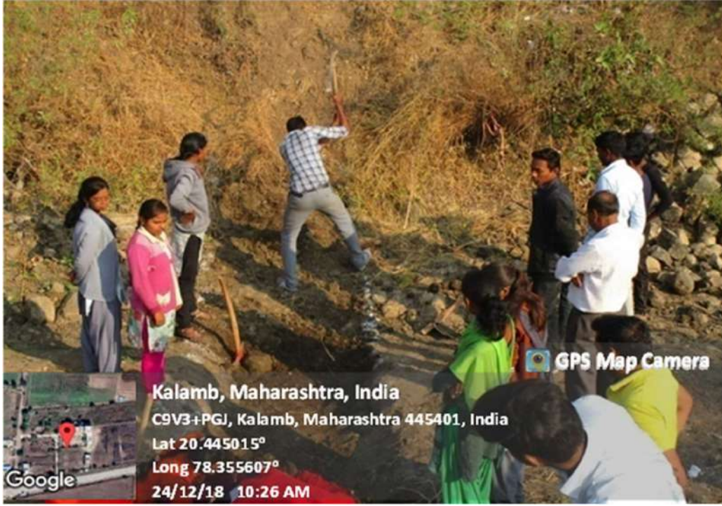
Snapshots During the Construction of Bund
